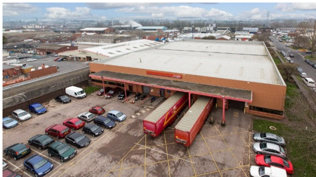
Exeter, 13 Trusham Road, Marsh Barton Industrial Estate
